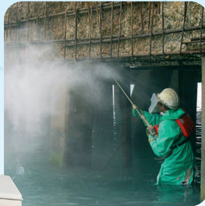
Concrete cutting - 1000 bar
