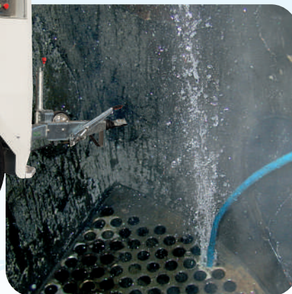
Heat exchanger cleaning - 800 bar
