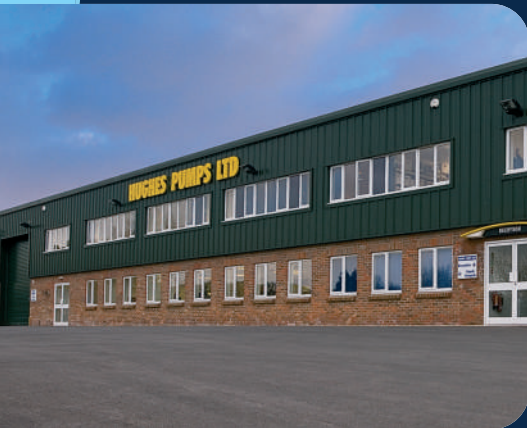
New Hughes Pumps factory constructed in 2004
